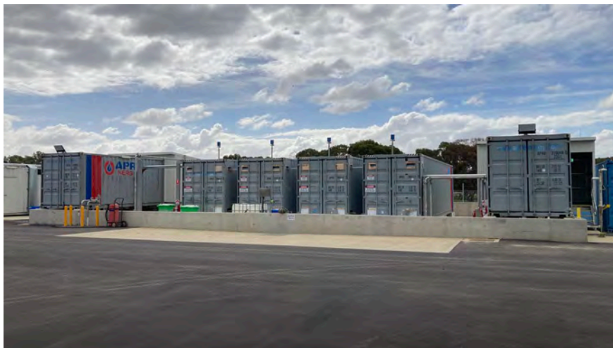
Figure 8: View of the Tanker Unloading Bay and Sump
