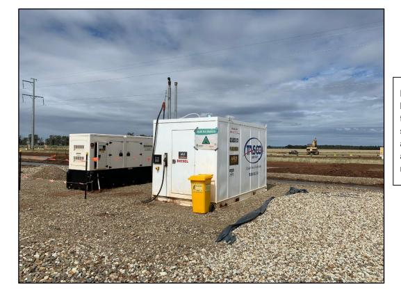
Plate 6: View of the site bunded fuelling area at the time of the auditor's site visit on 02/03/22. An appropriately stocked and secured spill kit was noted to be present.
